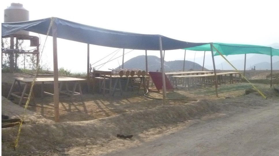
Figure 12 – Core Farm ready for drilling.
