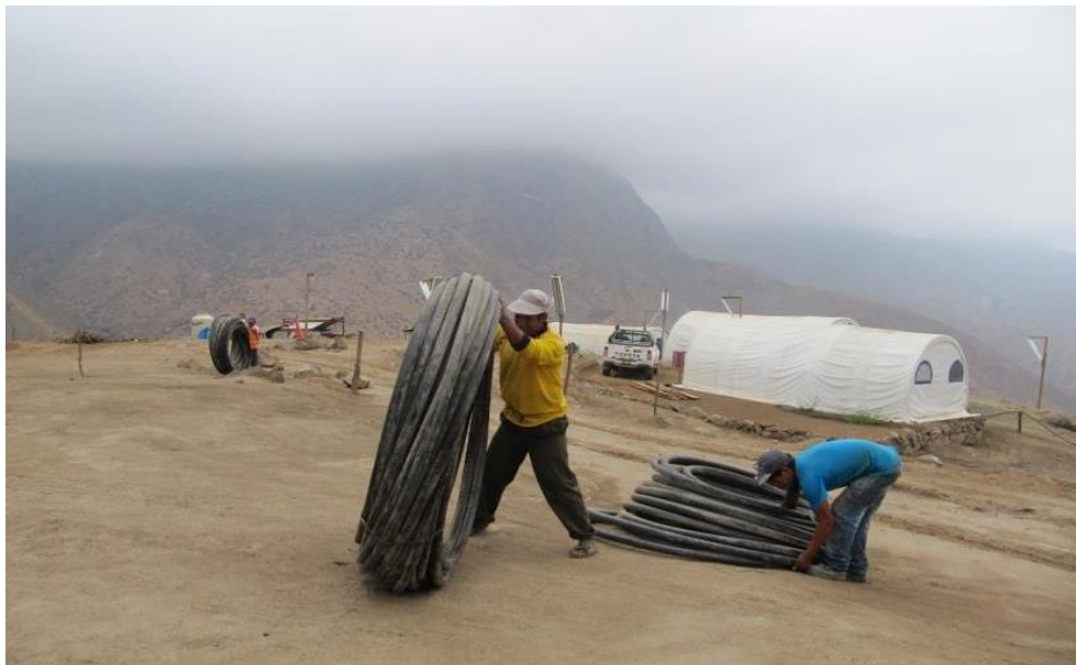
Figure 11 – Preparing waterlines for drilling.
