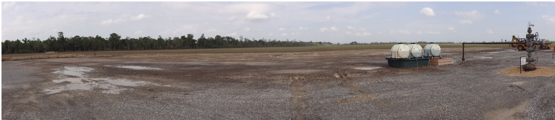
Site of Rosewood Plantation 21H with well head on the right hand side and flare stack in the distance to the left
