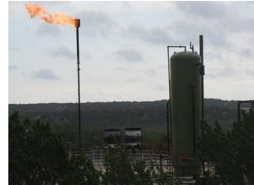
Production facilities on the Devon Bishop 1H Cline Shale well
