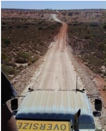
Access road sheeted
