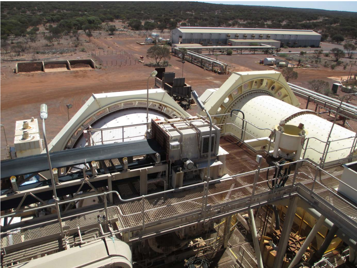
Figure 8: Thunderbox SAG & Ball mills with the dual fuel powerstation in the background
