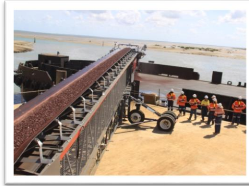
Bing Bong Loading Facility
