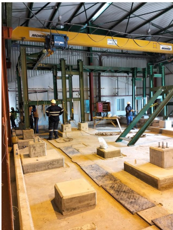
Figure 3: Drying and Packaging – Plinths and foundations ready for structure and calciner installation
