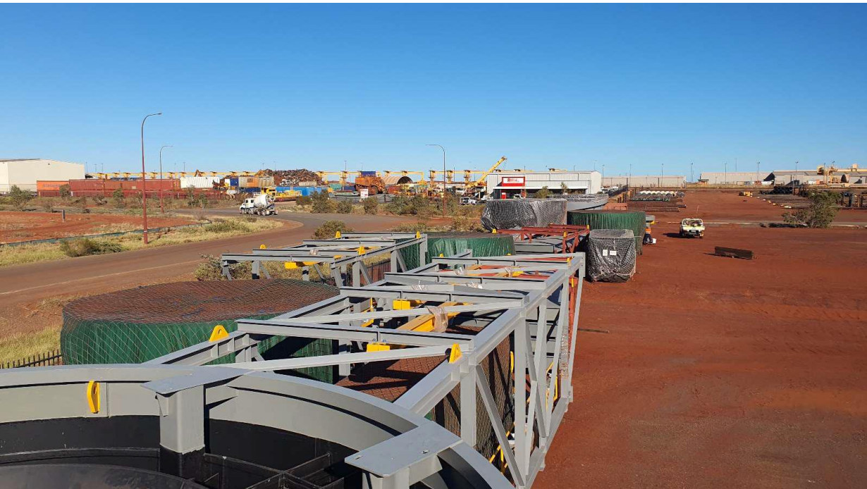
Flotation Cells & Structural Steel ready for installation.
