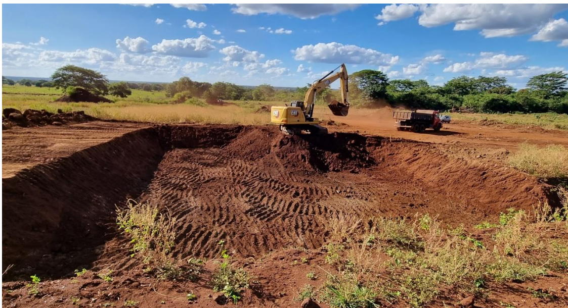
Figure 4. Trial pit excavated by vendor EDEM in May 2023; upper part of alkaline complex is very weathered and suitable for free digging by excavator.
