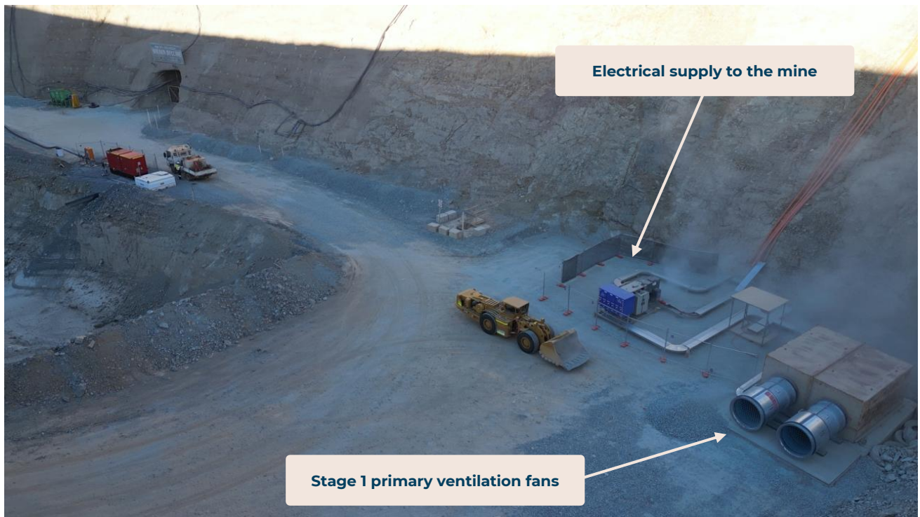
Figure 5: Power and mine services established to the Andy Well underground. Stage 1 primary ventilation also installed in advance of first ore development in mid-2025.
