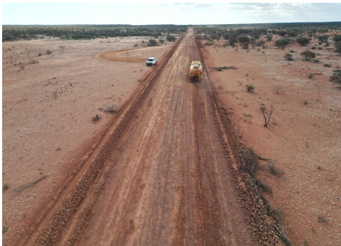
Figure 8: New 20km haul road between the processing plant and the open pit mining area in anticipation of open pit mining fleet mobilising, January 2025.
