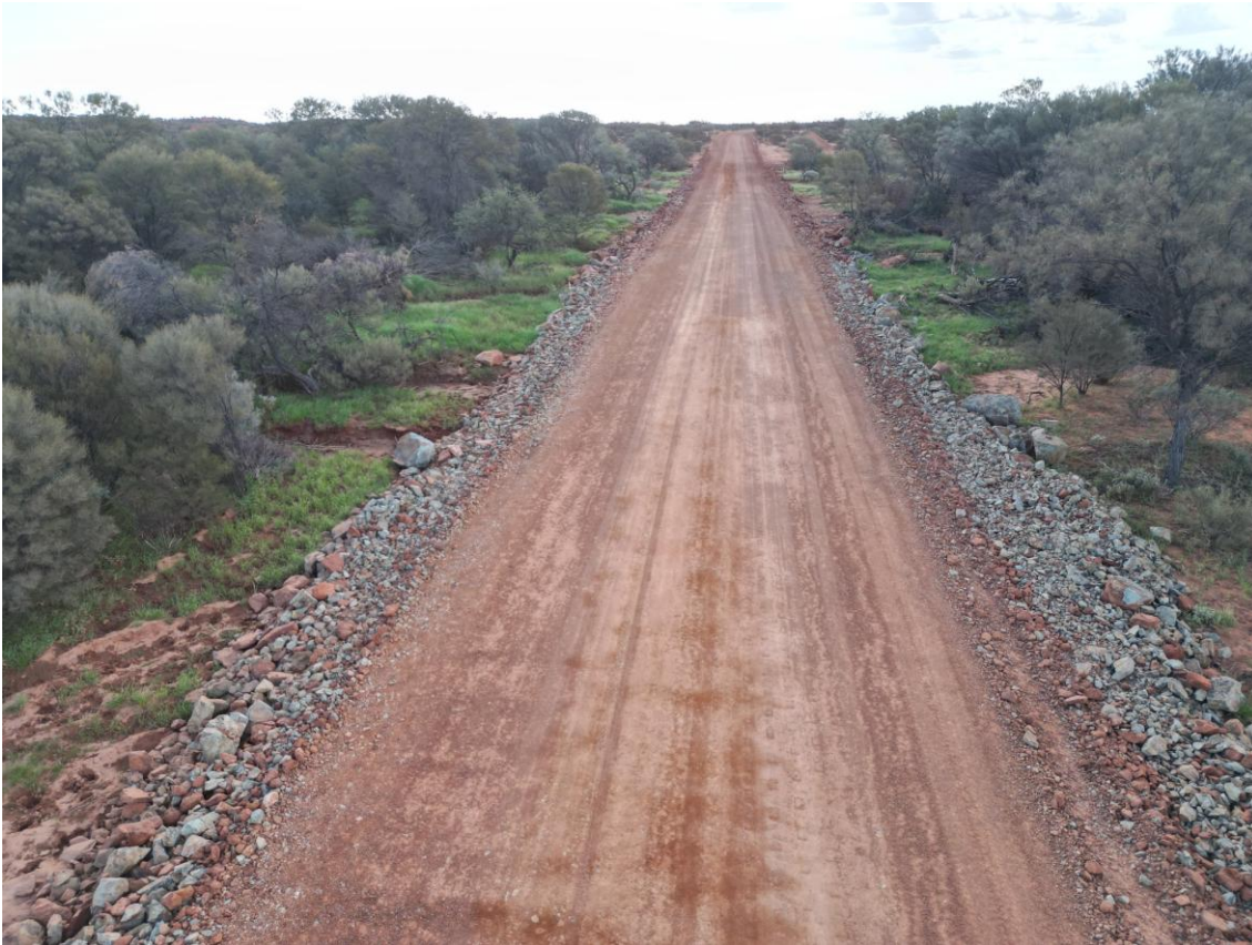
Figure 9: Example of upgraded section of haul road between the processing plant and the open pit mining area with rock armouring on shoulders to ensure long term resilience during wet weather events, January 2025.
