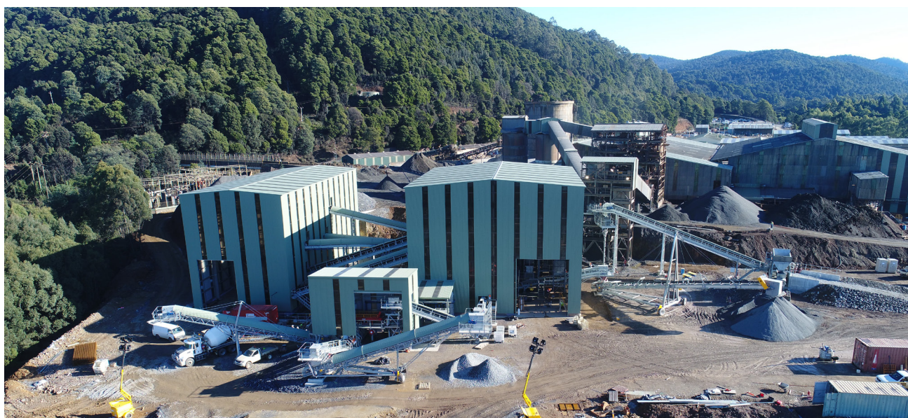
FIGURE 1: RENISON ORE SORTER SHOWING NEW BUILDINGS HOUSING THE CRUSHER (LEFT) AND THE ORE SORTER (RIGHT)
