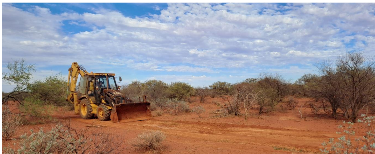
Image 1: Drill pad preparation in progress at Yanrey
