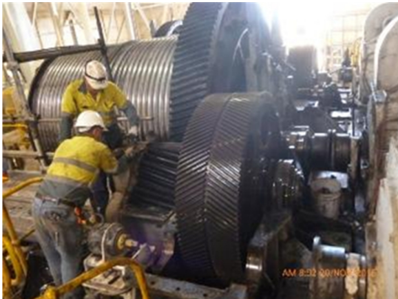
Removing hoist gearing
