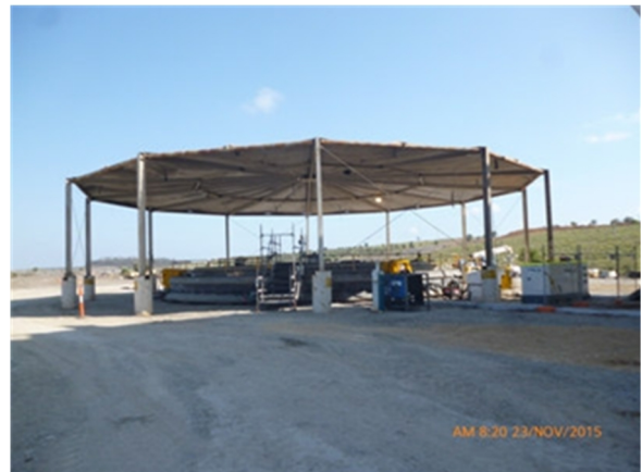
Tent over tub for swing rack installation
