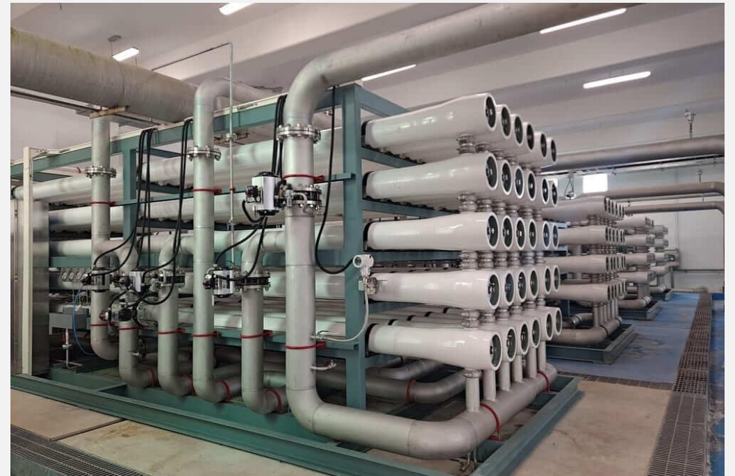
EXAMPLE OF A SKID MOUNTED NANOFILTRATION PLANT 2
