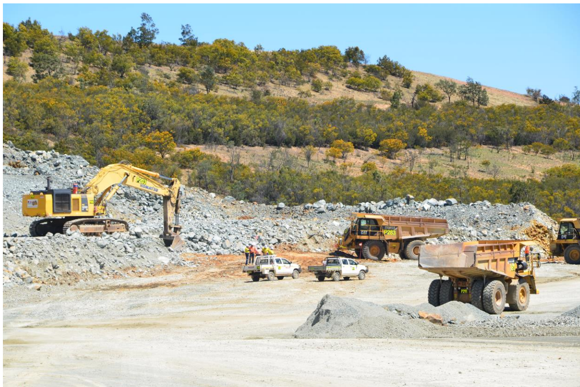
Figure 4: Clearing of underground box cut area
