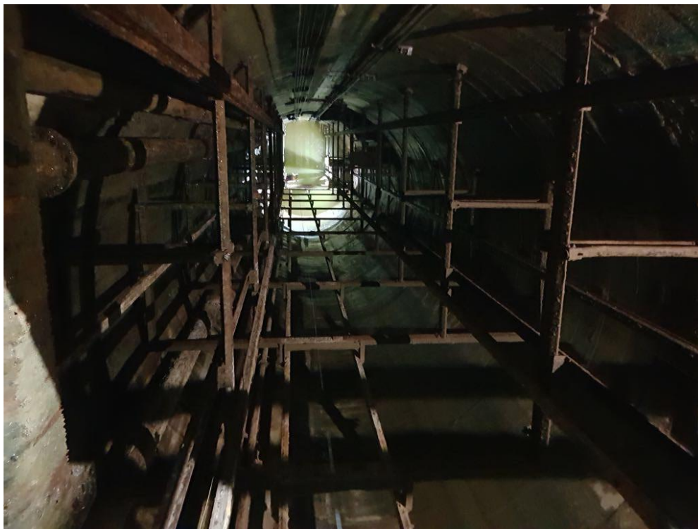
Figure 3: (Top) Plan-view schematic showing the configuration of the Hutchings Shaft and (Bottom) photograph of the Hutchings Shaft taken in January 2018 showing a similar plan-view perspective, with the accumulated water at the 350m Level.
