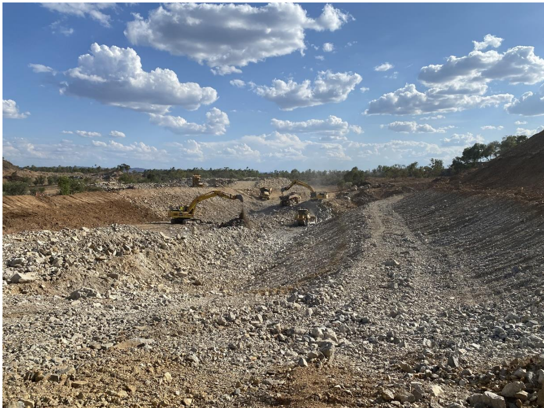
Figure 3: Wisles Dam – Embankment Works
