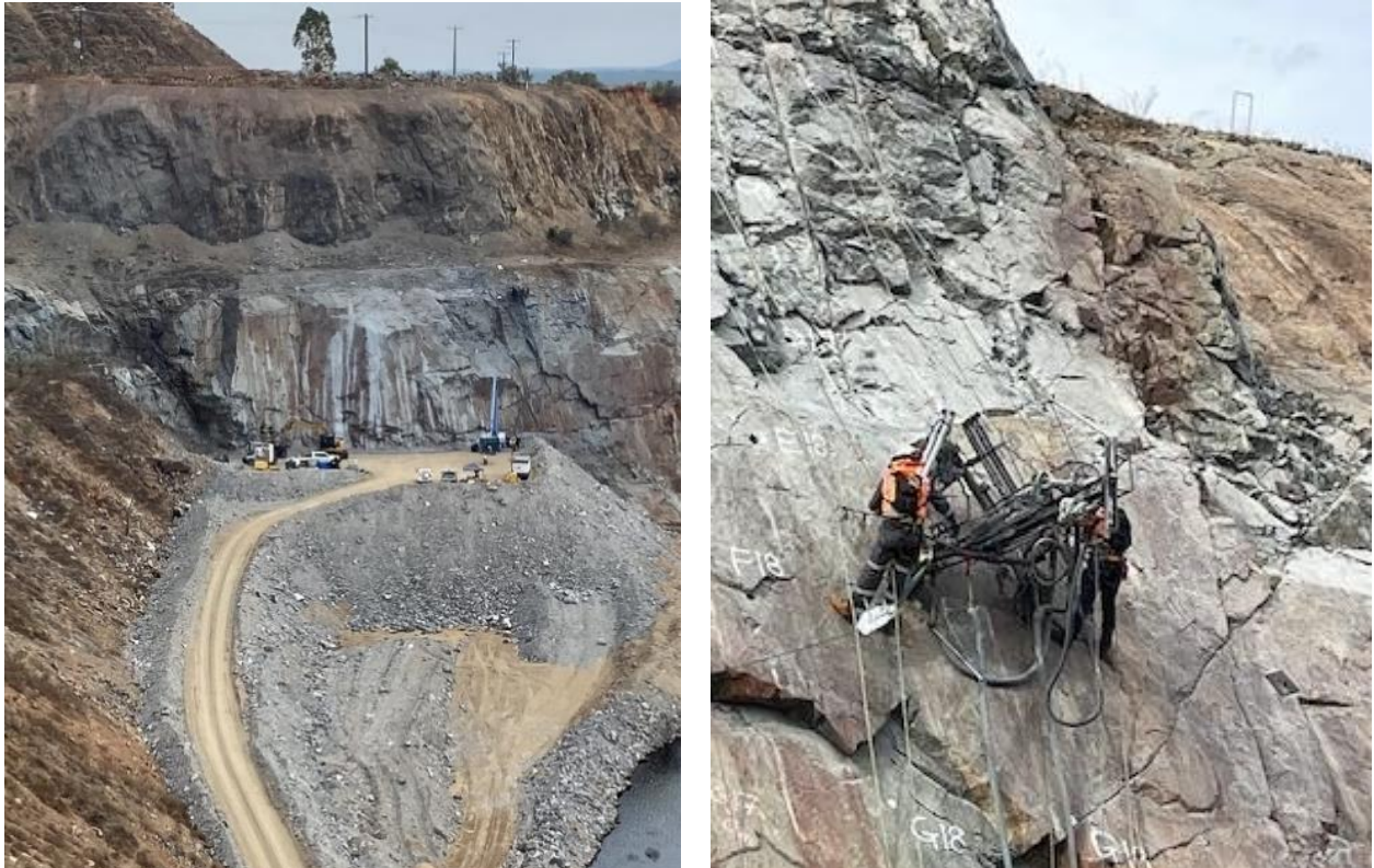
Figure 2: Drilling works ongoing for MAT Face Stabilisation
