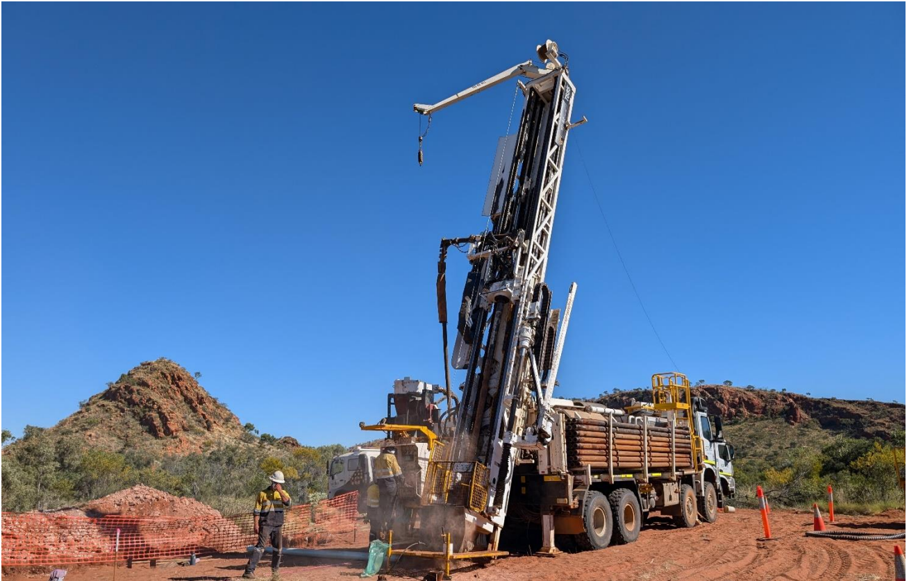
Figure 1: RC Drilling begins at Bigrlyi with the collaring of Drillhole BRD2401
