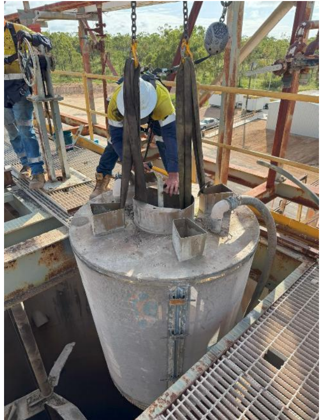
Area 03 – Removal of CIL intertank screen
