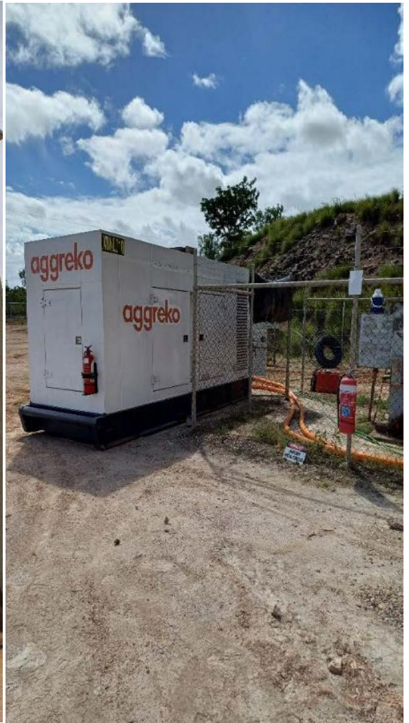
Generator in position and terminating of 300mm 4core and earth cables at Area 01
