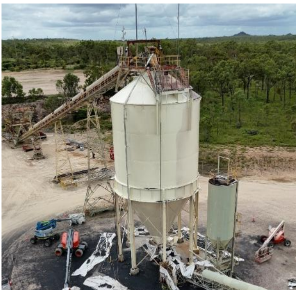
Remedial works, blast and paint of fine ore bin and reagent tanks - April 2025
