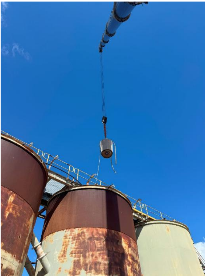
Area 03 - Lifting of CIL intertank screen
