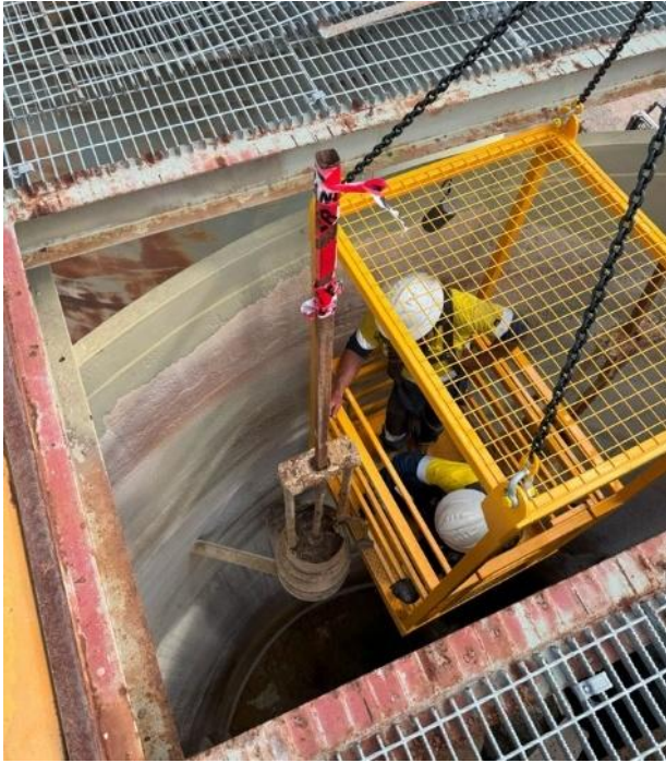
Area 03 - CIL tank intertank screen support structure removal
