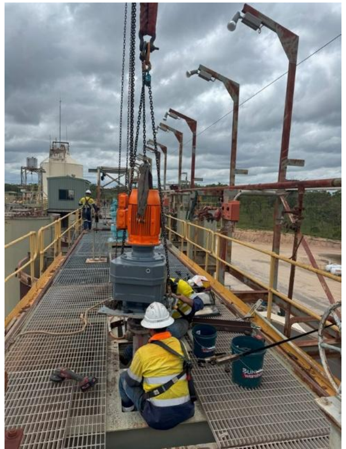
Area 03 - Installation of new CIL agitator gearbox
