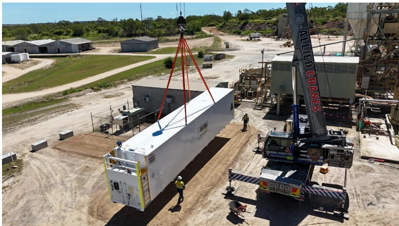
Figure 1: Lifting and installation of NMR 100kL self-bunded fuel tank
