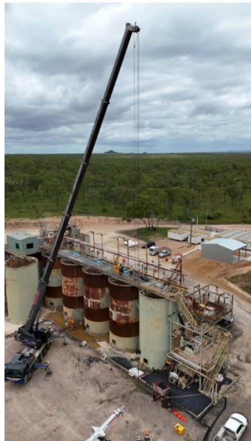
Area 03 - CIL tank intertank screen, gearbox & agitator works
