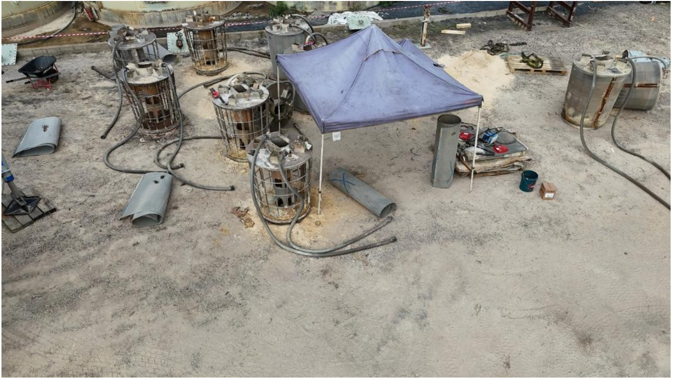
Area 03 - Refurbishment of CIL intertank screen
