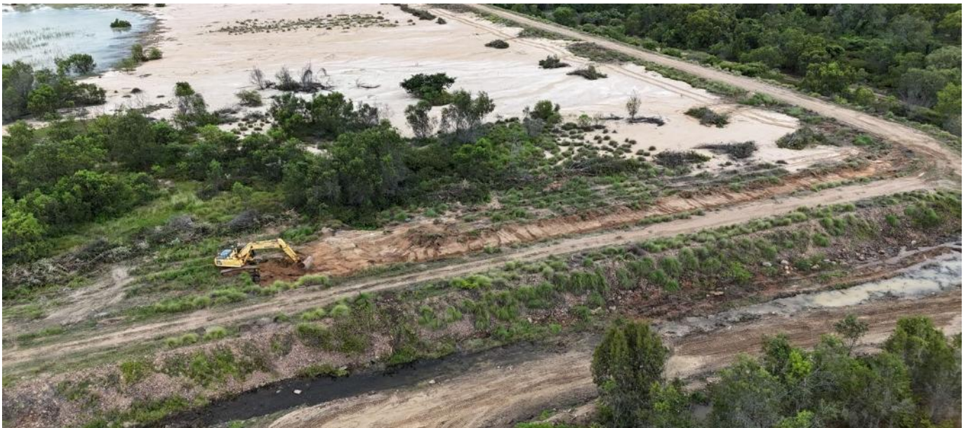
TSF maintenance earthworks on north embankment (Northern Cell)
