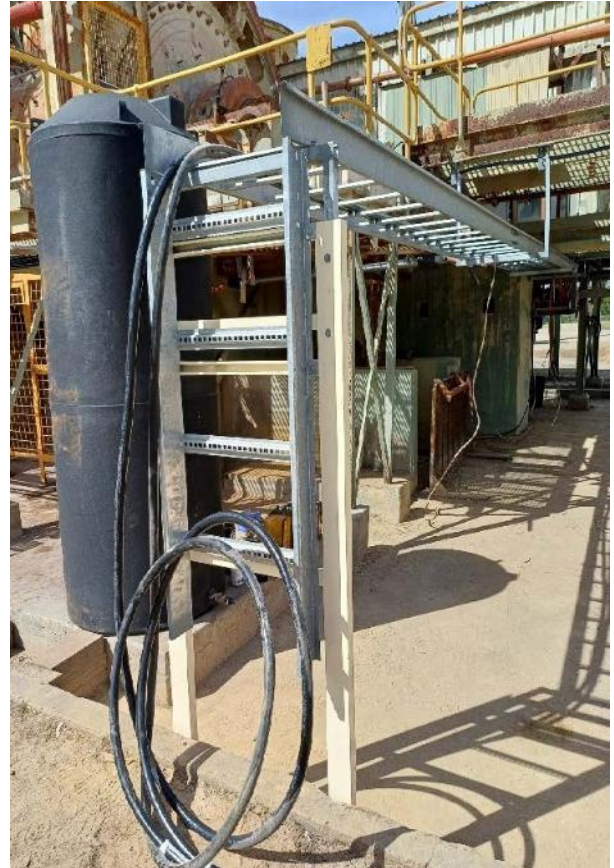
Area 02 - Installation of cable supports and cable ladder under ball mill discharge
