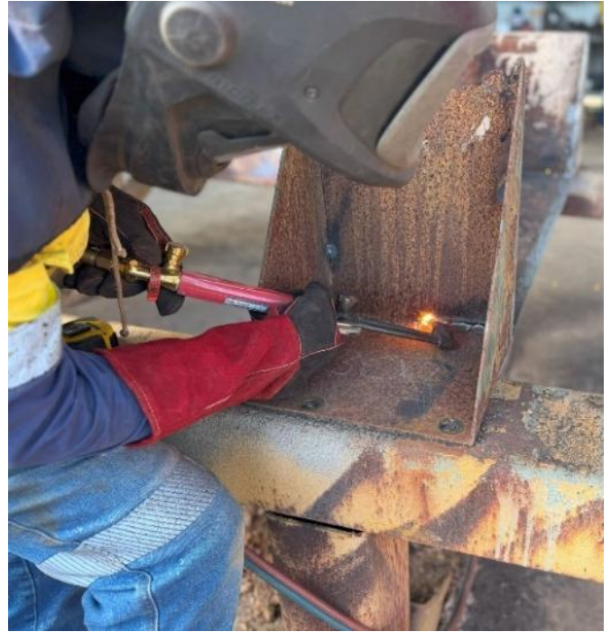
Area 03 - Repair works on 03-SN-13 launder box
