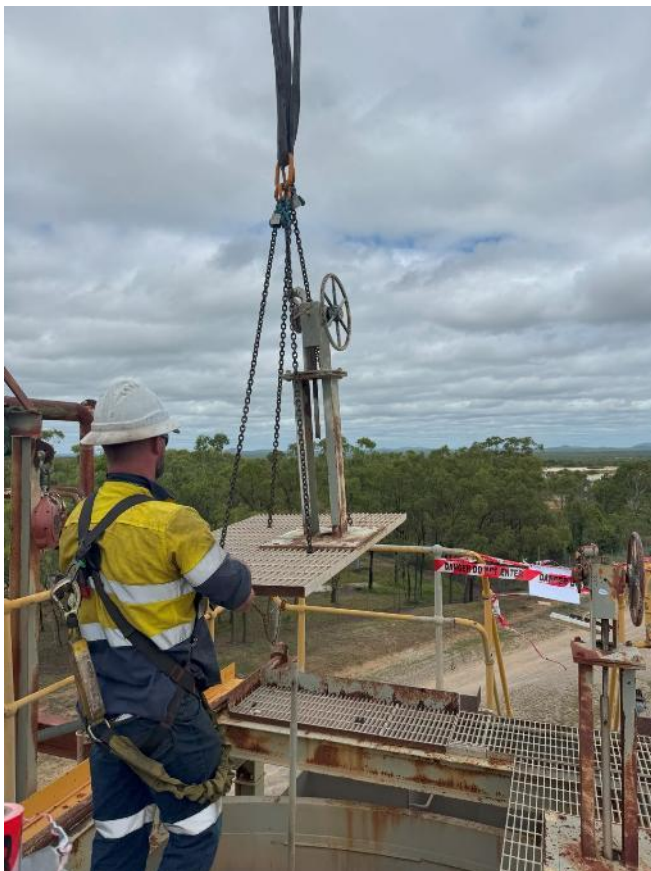
Area 03 - Remove wind up plug and spiral for service and repair
