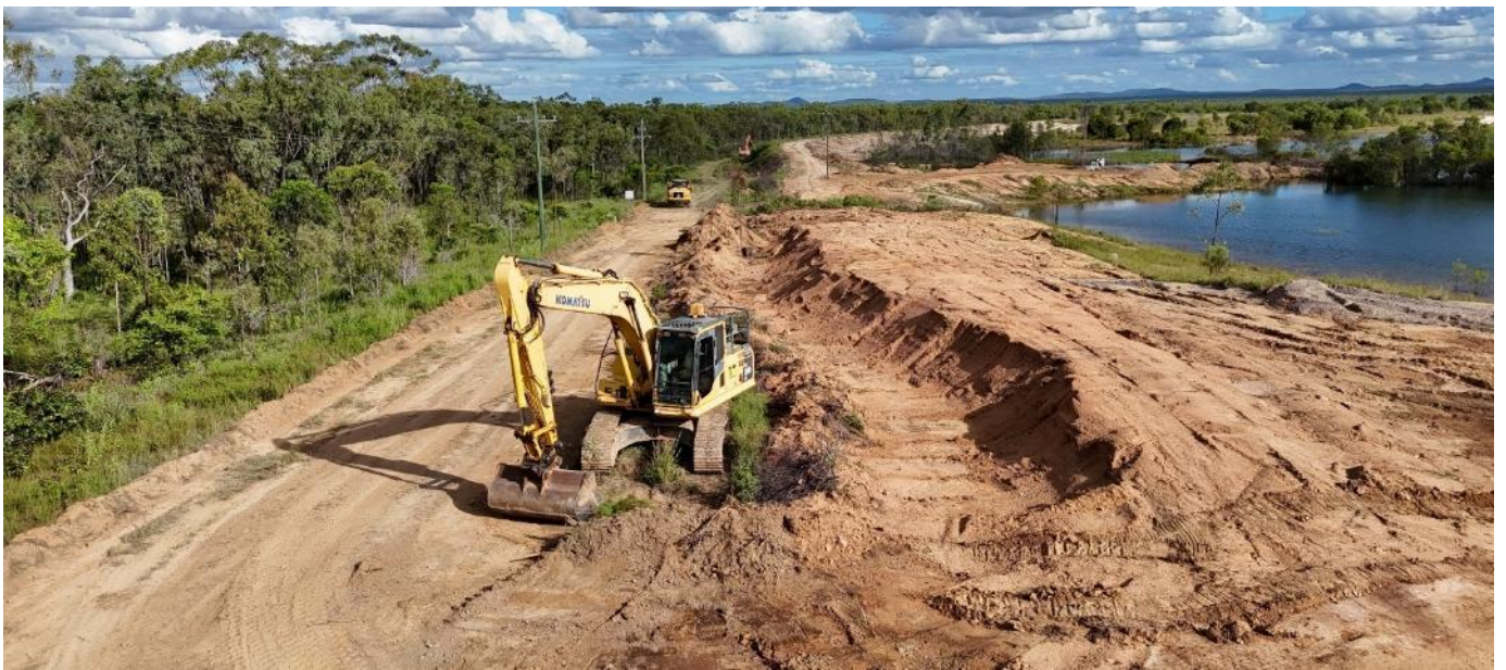
TSF maintenance earthworks on east embankment (Northern Cell)
