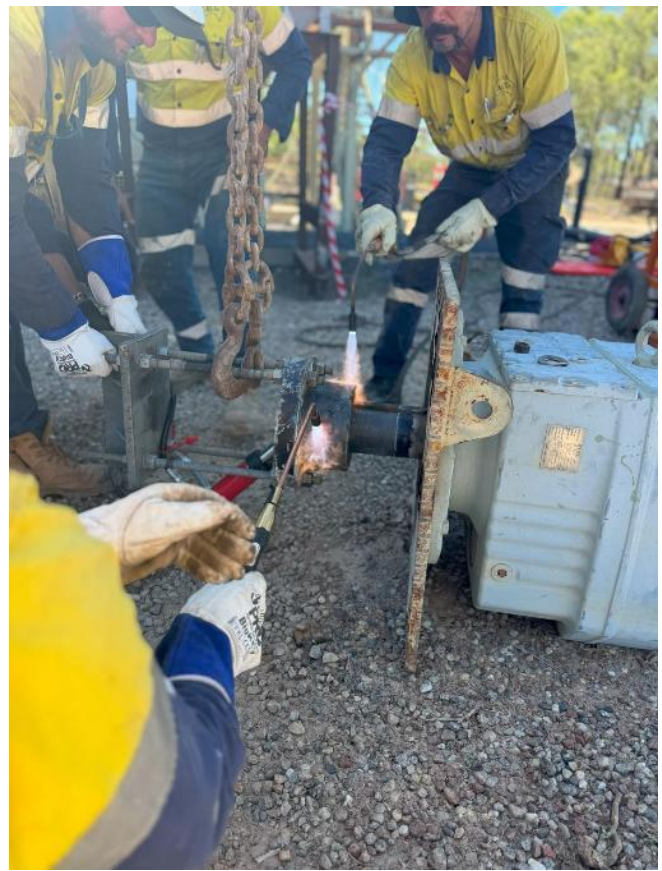
Area 03 - Remove coupling from old gearbox to install new gearbox
