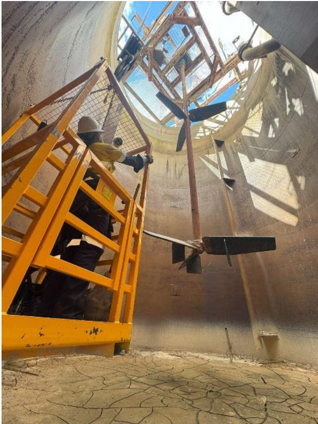
Area 03 - CIL tank damaged agitator blade changeout and reline
