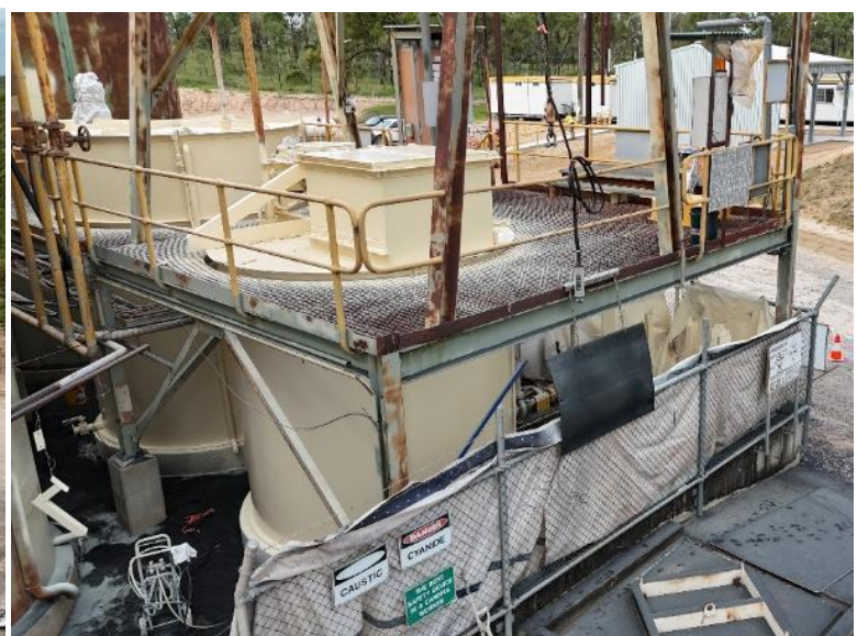
Remedial works, blast and paint of fine ore bin and reagent tanks - April 2025
