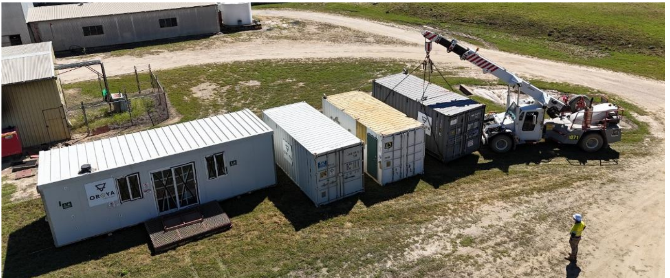
Laboratory container temporary positioning for installation in May
