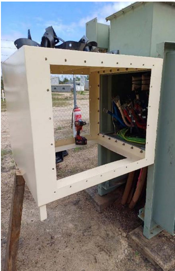
Area 02 - Marshalling box for generator installed
