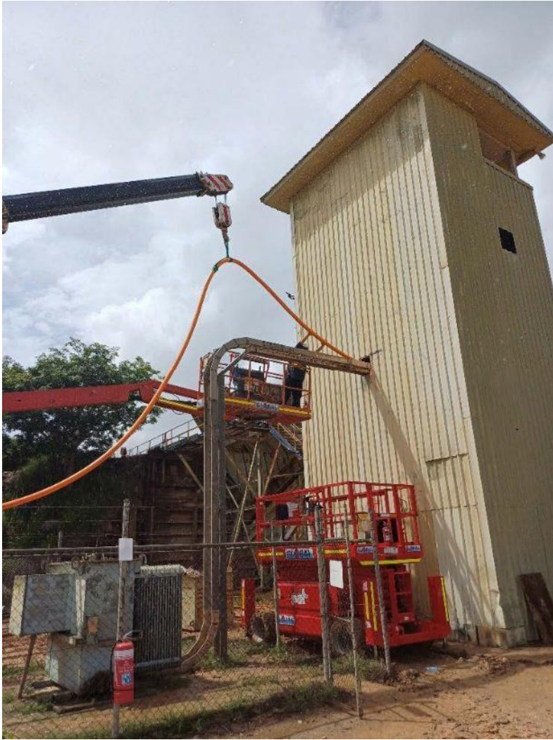
Generator in position and terminating of 300mm 4core and earth cables at Area 01
