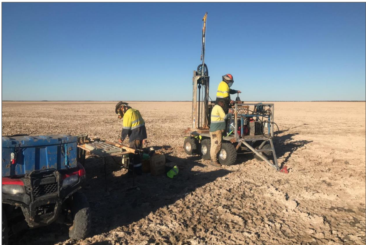
Figure 4. Sonic Drilling in Progress
