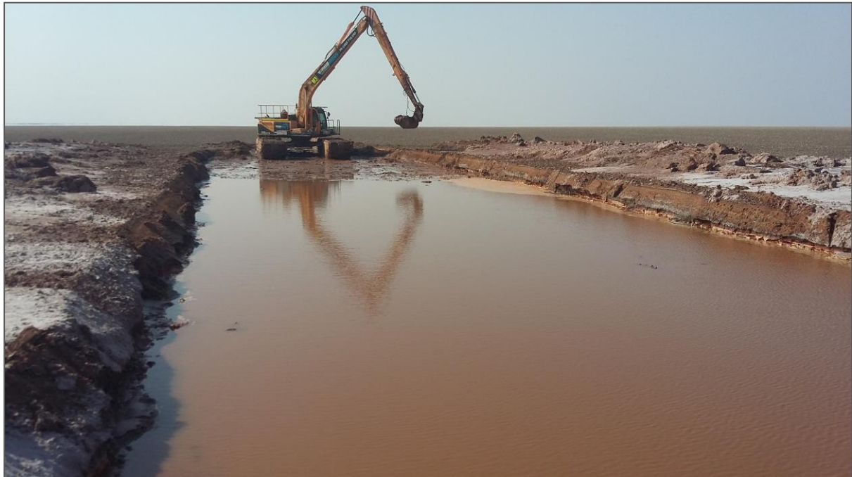
Figure 1. Trench Excavation in Progress
