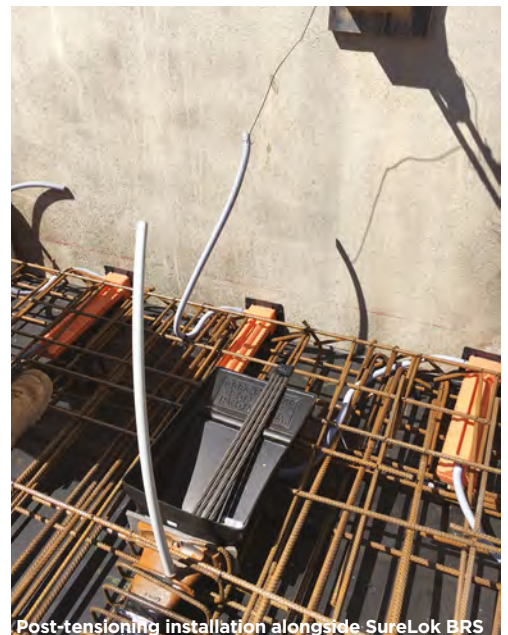
Post-tensioning installation alongside SureLok BRS
