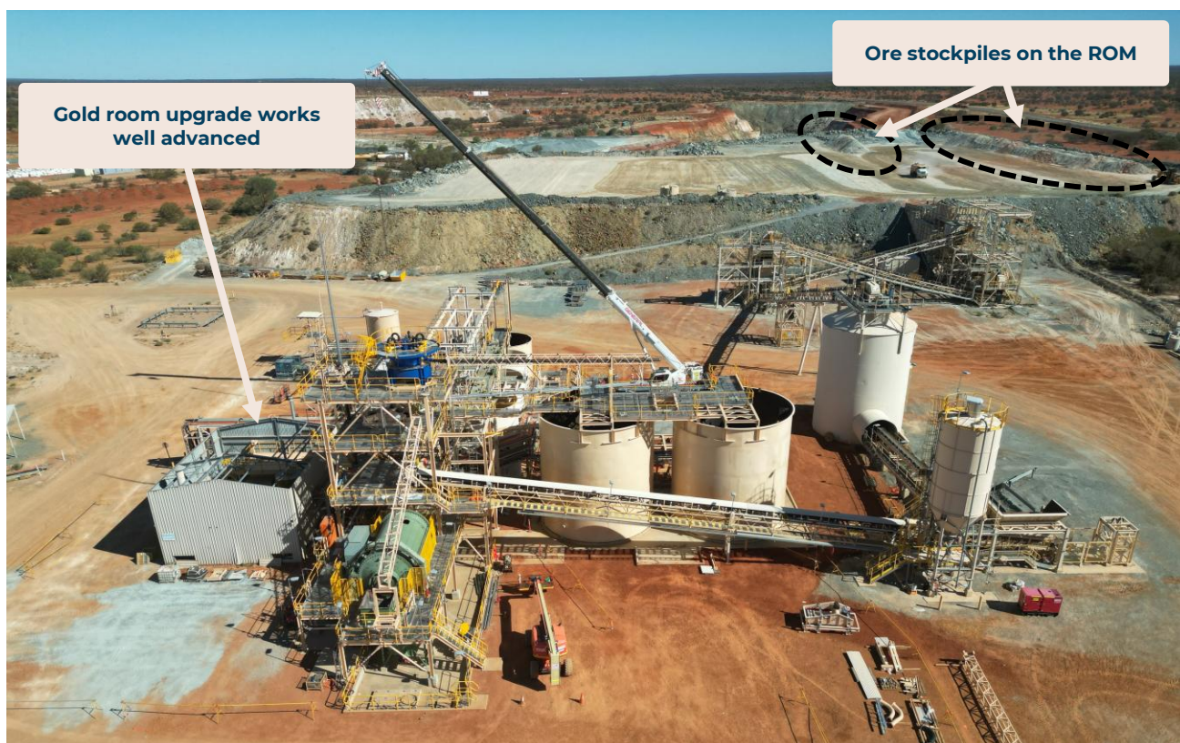
Figure 3: Major structure works completed at the process plant and focus now on gold room upgrade, note ore stocks on the ROM in the background, April 2025.
