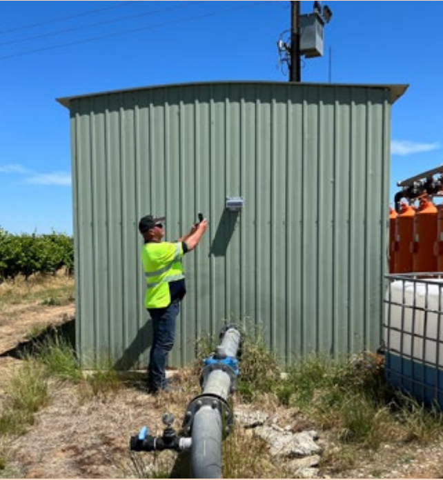
Entering a meter reading into the smart meter online portal to validate a smart meter installation.
