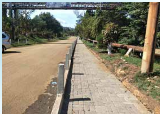
Pemanfaatan POTON (Pomalaa Beton) sebagai paving blok di UBP Nikel Sulawesi Tenggara. Utilization of POTON (Pomalaa Beton) as a paving block at Southeast Sulawesi Nickel Mining Business Unit
