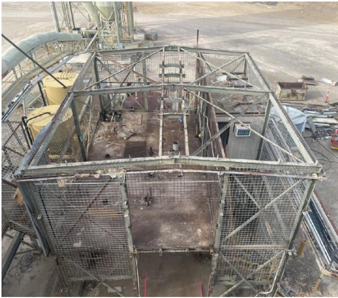
Start of floor removal from gold room upper level
