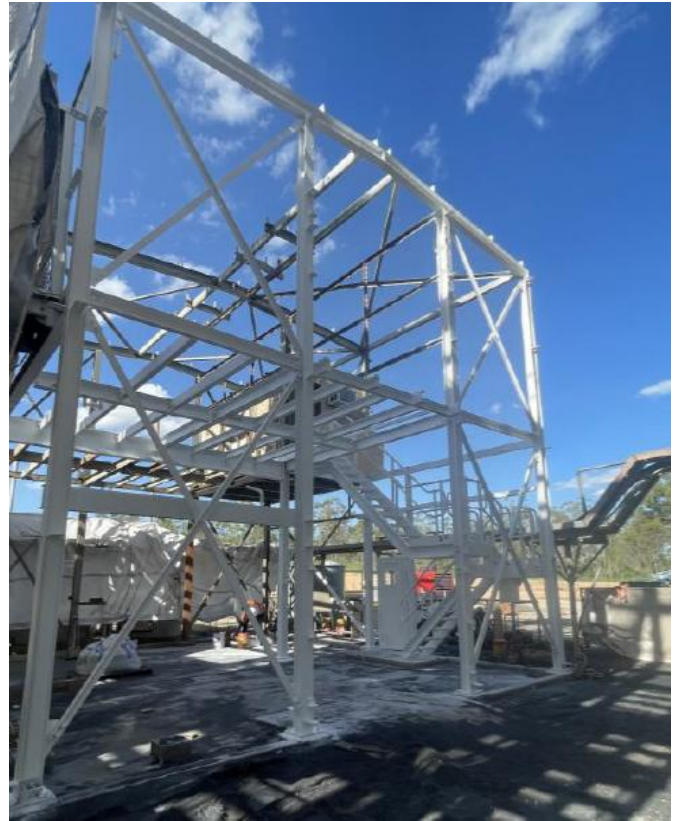
Putting second coat of undercoat on gold room structure
