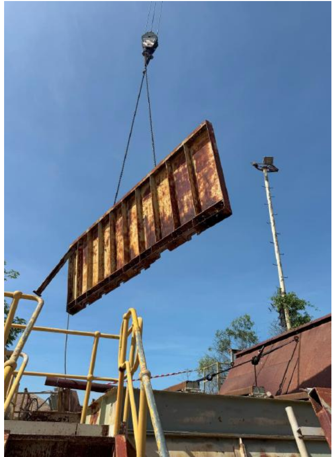
Rom Bin Wing Walls removal
