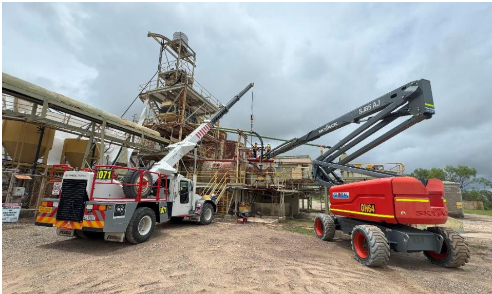
Figure 1: Refurbishment of Blackjack grinding area underway
