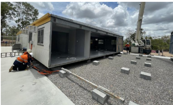
New Office block being placed and aligned
