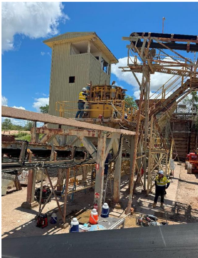
Cone Crusher removal and inspection
