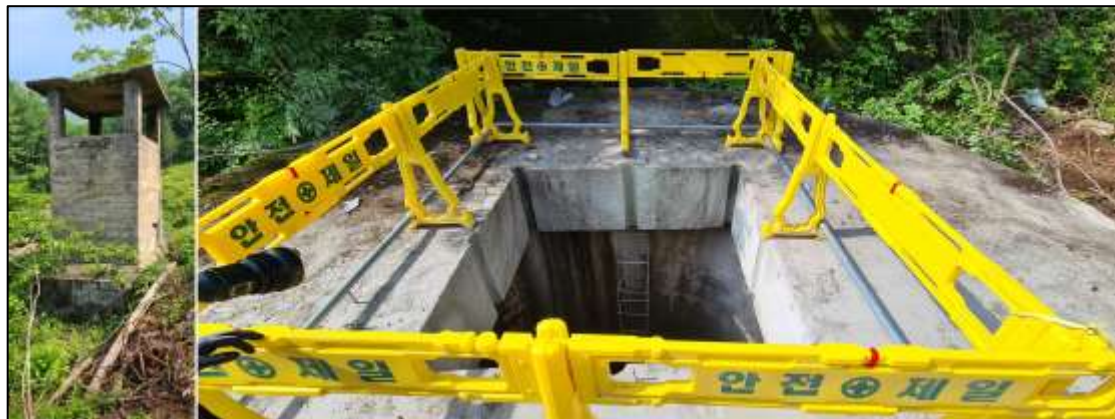
Figure 18-16. Ventilation Shaft Surface Openings
