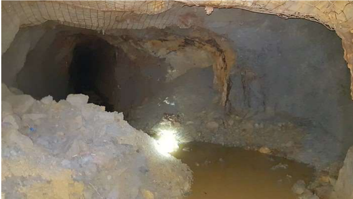
Figure 3 - Muck pile and face following the initial blast on the Keillors 8A Incline
