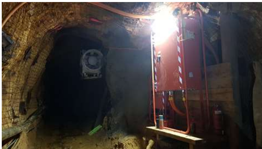
Figure 1 - The auxiliary fan and controls in place in No 8 Level Drive
