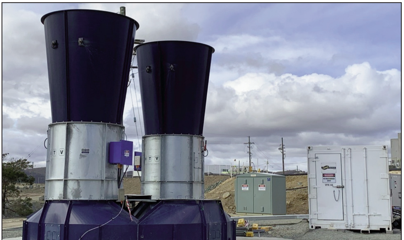
Figure 5: New vent fans installed for underground operations
