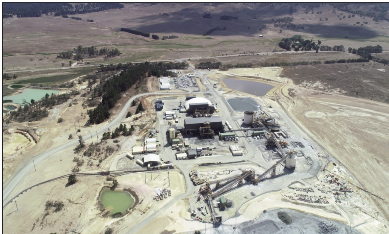
Figure 2: Woodlawn Processing Plant, with ROM Pad, crusher and fine ore bin in the foreground
