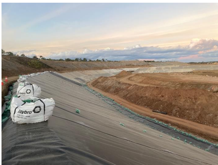
Figure 5: Wises Dam liner placement
