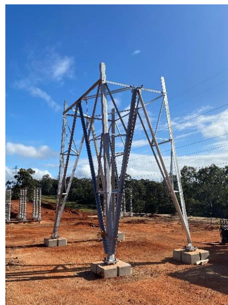
Figure 3: Lattice tower erection
