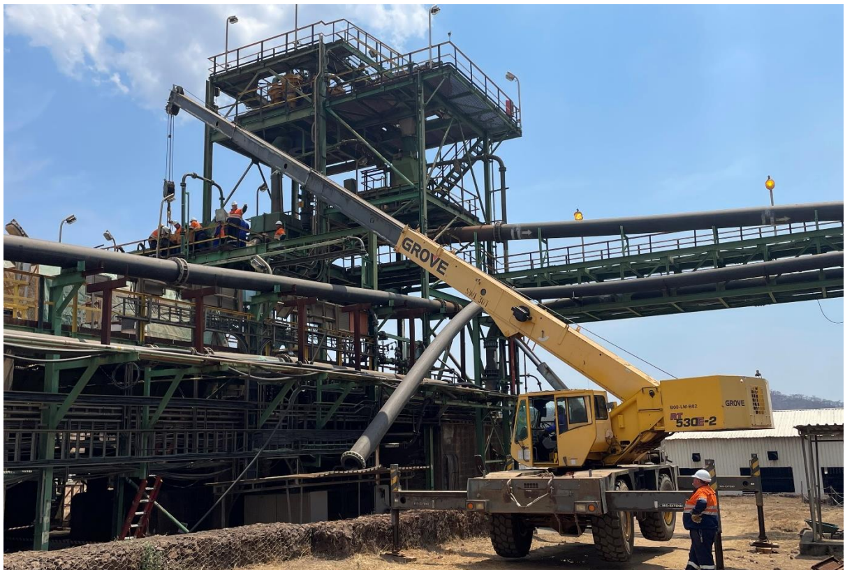
Figure 3: Feed conveyor gearbox repairs
