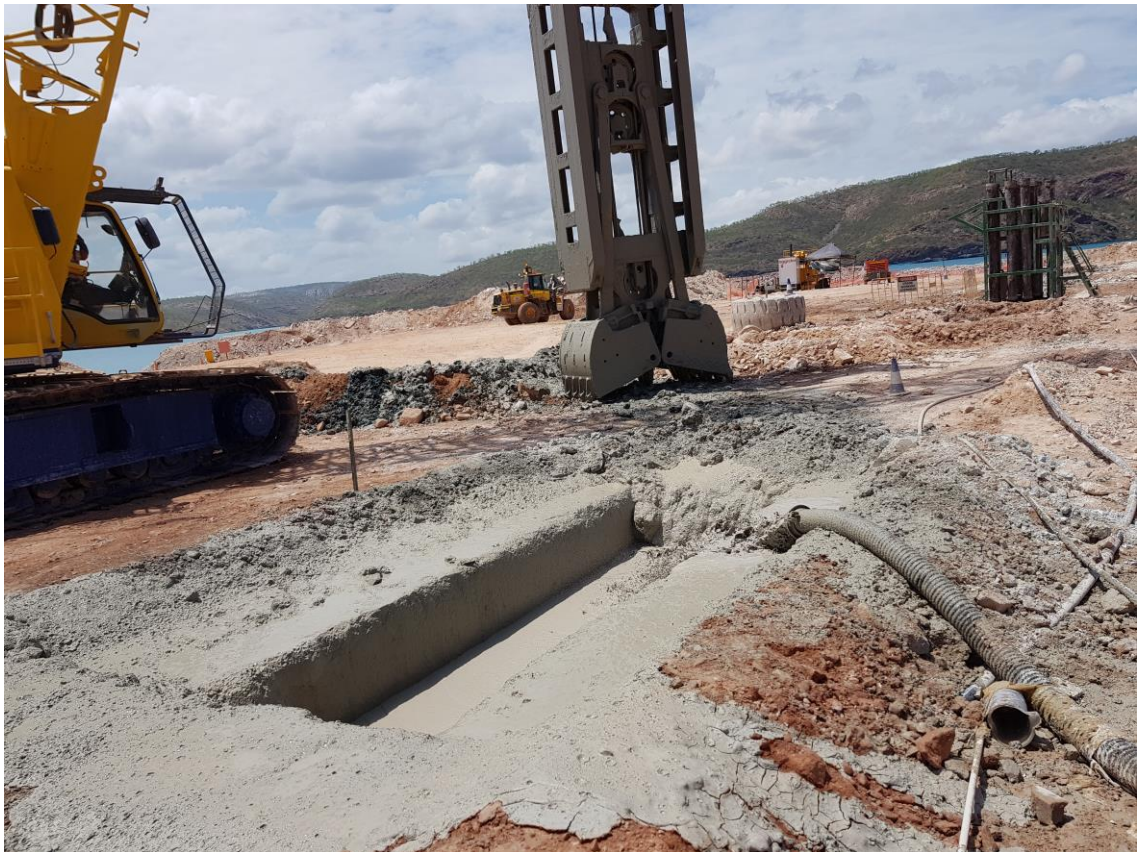
Figure 6: Pumping slurry into excavated Panel 011 December 2017
