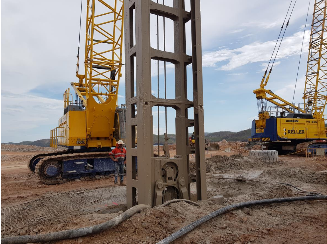
Figure 4: Excavation of Panel 016 - December 2017
