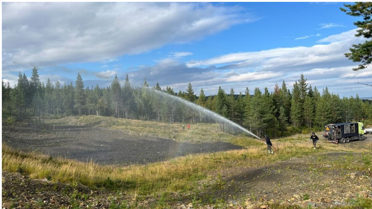
Figure 3 Moss priming application at the Nunasvaara South and Niska trial mine areas.
