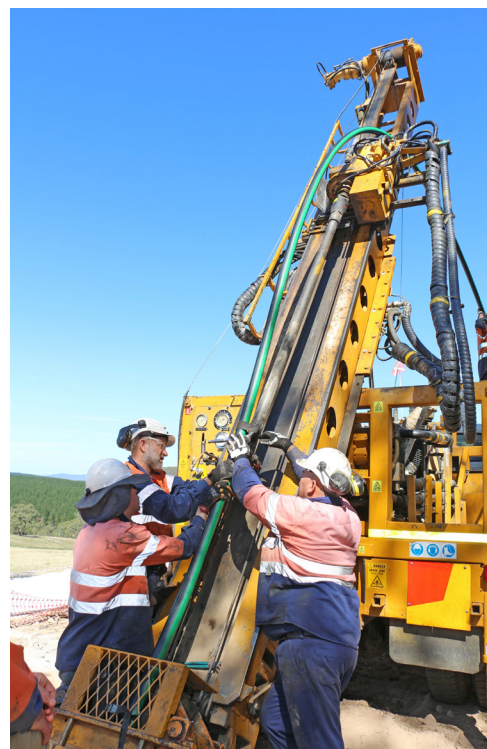
Figure 1 - The drilling crew completing the casing of Hole #1 with high pressure polyethylene pipe on Thursday 5 February.
