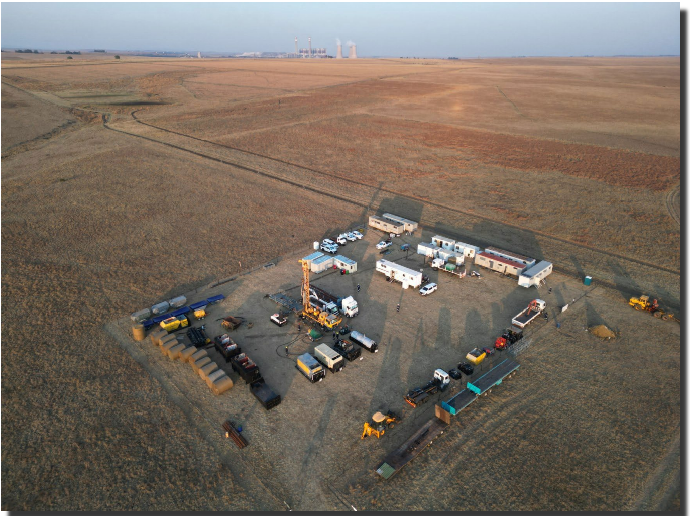
Figure 3: Production drilling rig on site for spudding well ER271-23PT with Majuba power station in the background.
