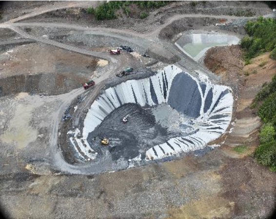
Veovača TSF Stage 1 complete and filling Stage 2 earthworks underway and Geomembrane installations begins shortly
