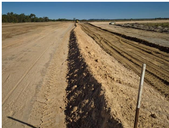
Northeastern wall subgrade finished
