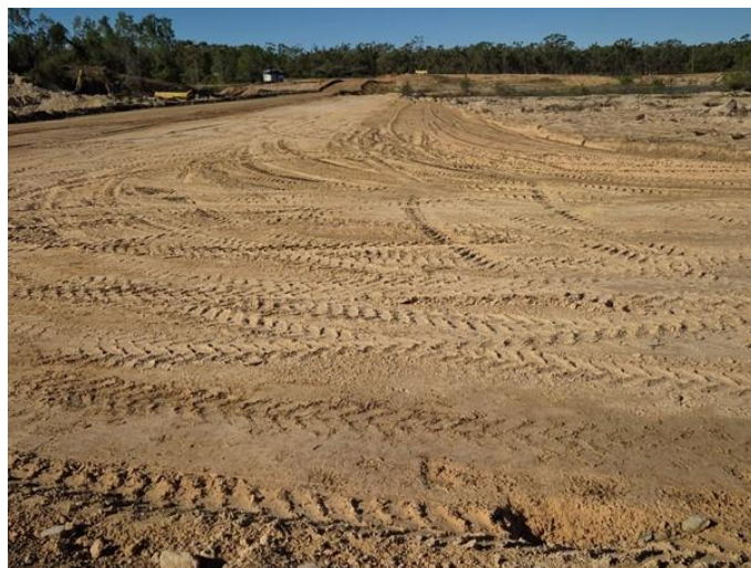
Northwestern wall subgrade finished
