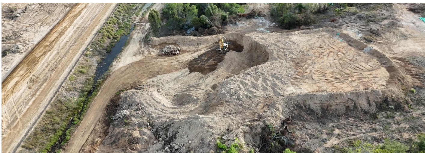
Mixing and blending gravel at Borrowed Area
