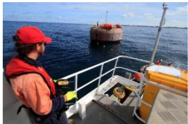
CETO Unit 2 prepared for deployment quayside along CETO Unit 3 (L), Carnegie operations team member controlling position of Buoyant Actuator from deployment barge (R)
