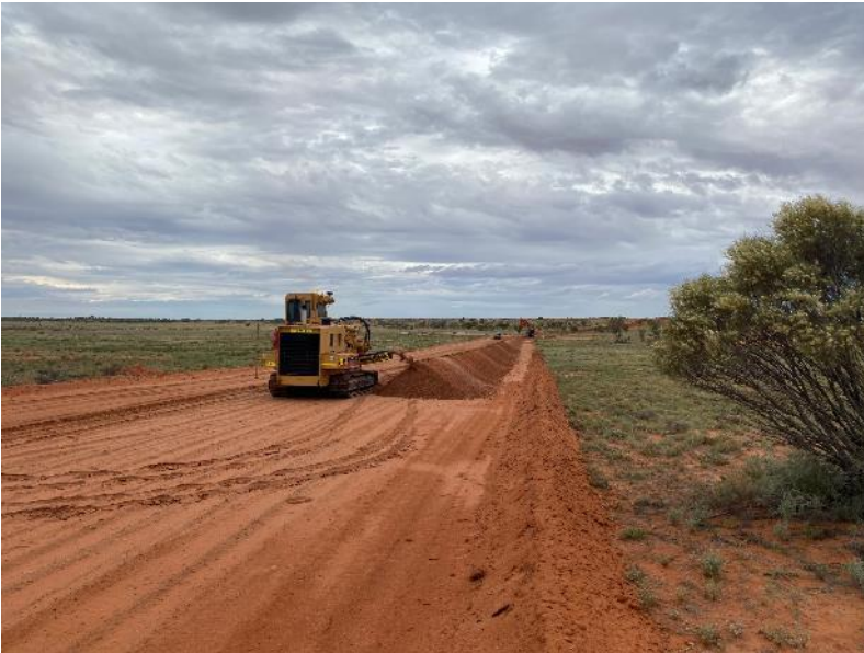
Trenching pipeline route from Vali
