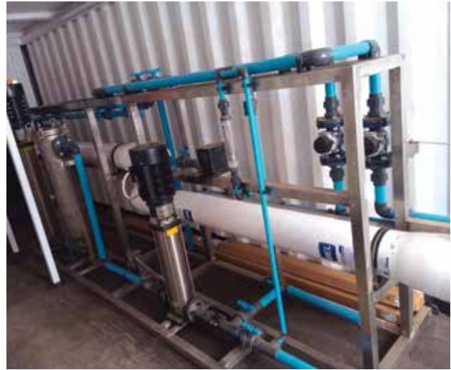
(Left) Water treatment pilot plant mobilisation. (Right) Commissioning the chemical treatment, filtration and reverse osmosis components of the pilot water treatment plant, setup to operate at 5m 3 /hr of feed water.
