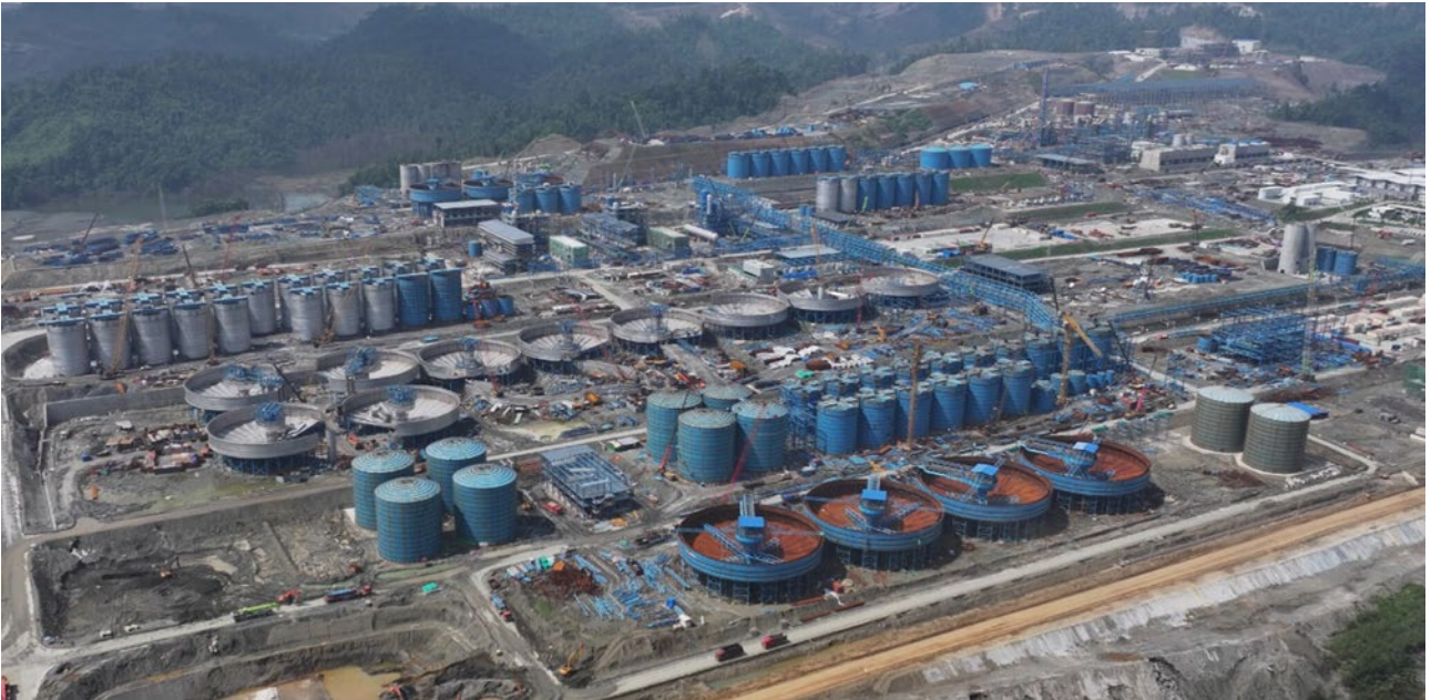
Main process equipment for ENC HPAL smelter: autoclaves, CCD, reactors and thickeners
