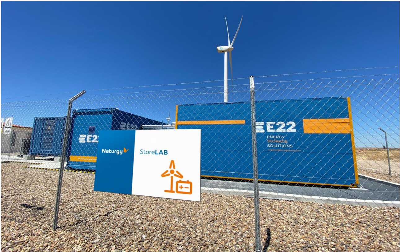
Figure 1 E22 250kW/675kWh VRFB installed in Zamora, Spain
