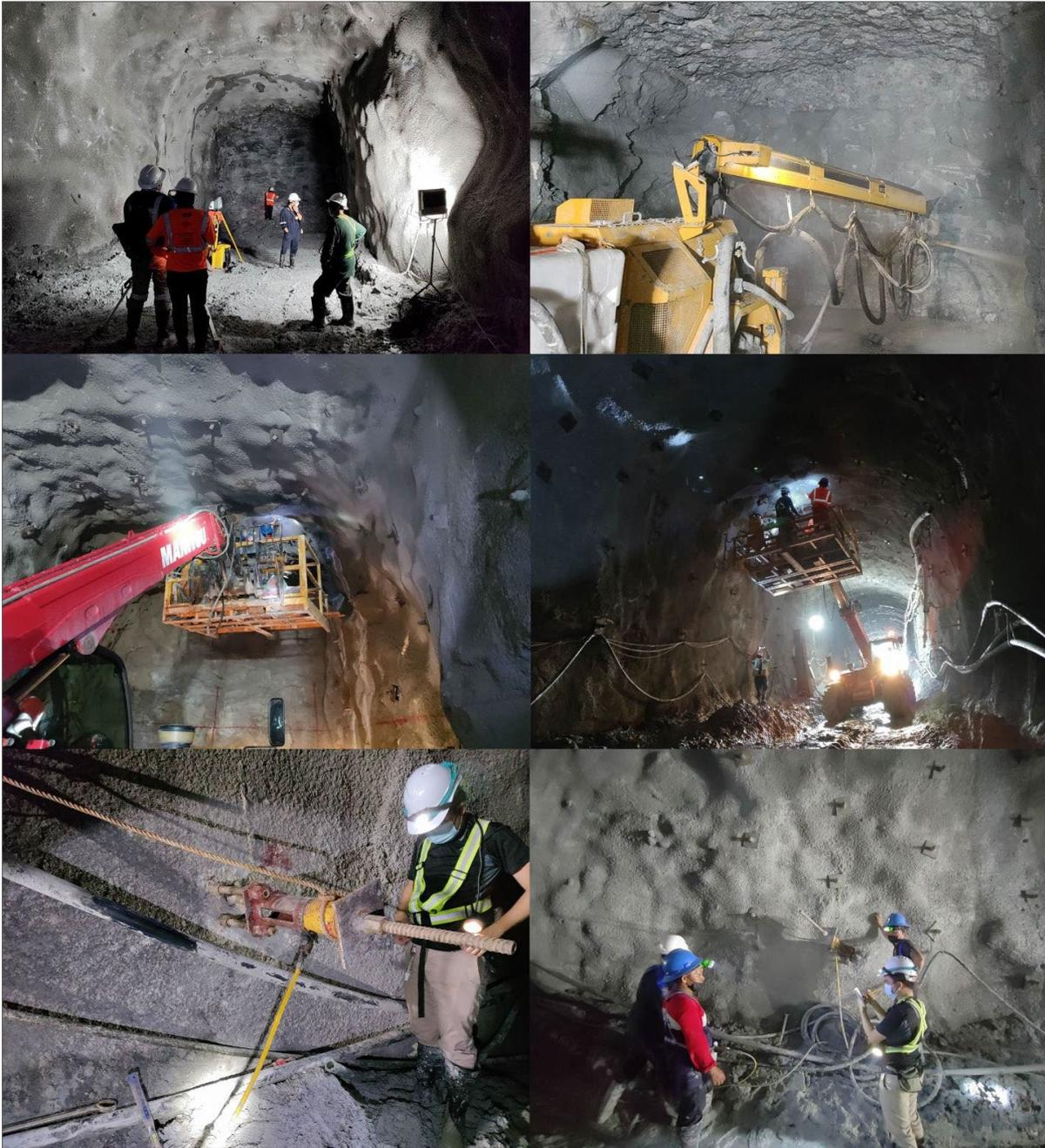
Photo 1: **Decline Development Cycle** - Face drilling & blasting, mucking, scaling, initial shotcrete spraying (batching), survey & mapping, rockbolt installation, final shotcrete spraying, and QAQC activities (Pull-out and thickness testing).
