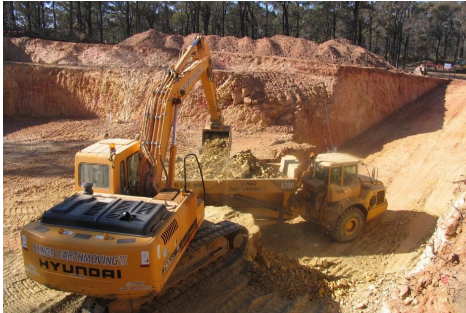
Figure 3: Excavating Bulk Sample Pit at Harvest Home
