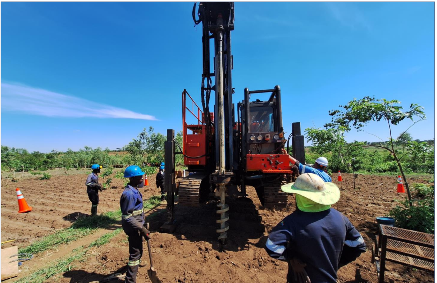
Figure 3: Auger Drilling
