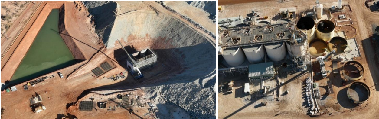
Figure 2: KoTH plant expansion project (crusher box cut excavation on left and tank erection progress on right)
