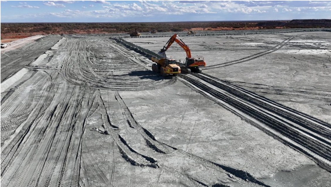
Figure 6: TSF lift underway, February 2025.
