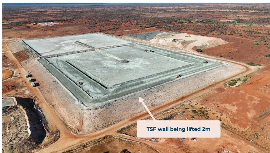
Figure 5: TSF lift underway, February 2025.
