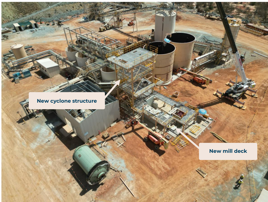
Figure 7: New cyclone structure and mill deck for the expanded processing plant, February 2025.
