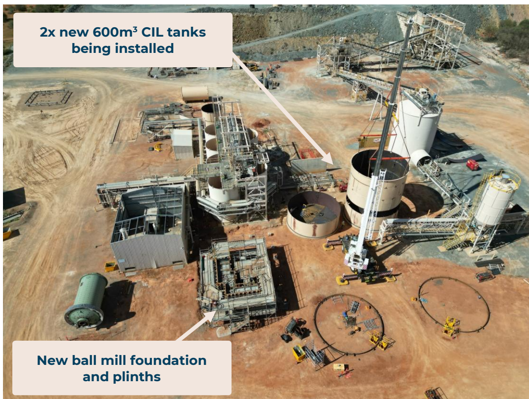
Figure 2: Drone image of the new ball mill foundation and plinths in the foreground and tank installation in the background, December 2024.
