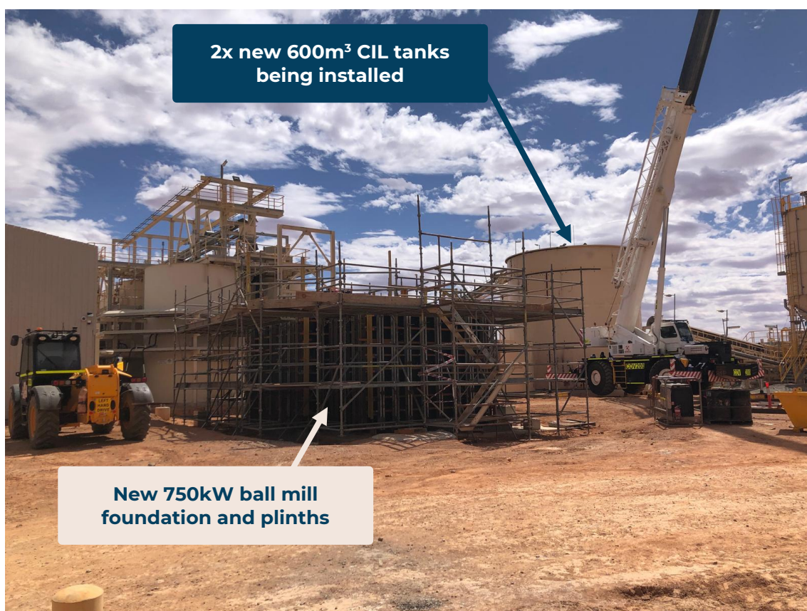
Figure 4: New ball mill foundation and plinths for larger 750kW ball mill, December 2024.
