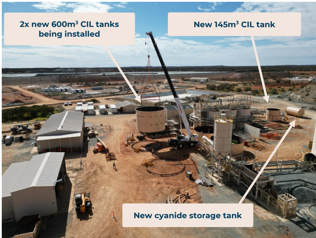
Figure 1: Drone image of the 2x new 600m³ tanks being installed for the expanded CIL circuit, December 2024.
