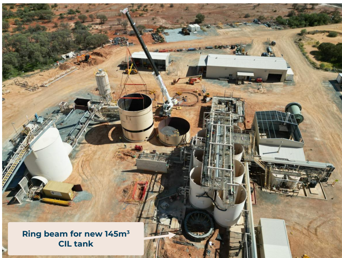
Figure 3: Drone image of tank installation, December 2024.
