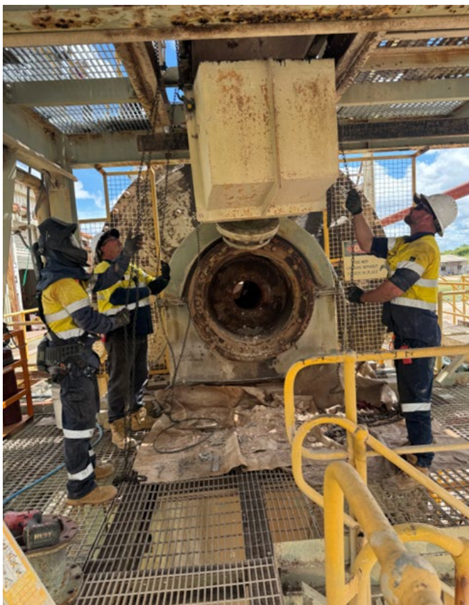
Area 02 ball mill feed end chute repair
