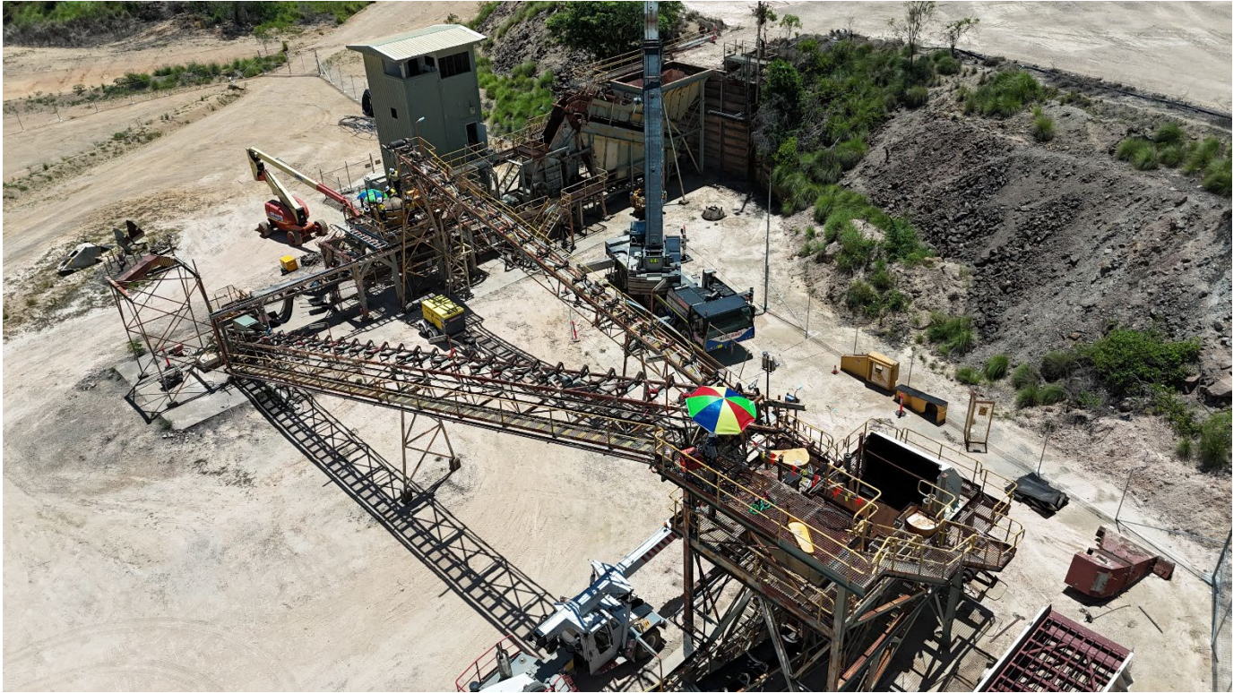
Area 01 with all conveyors belt removed for new pulley, bearing, roller, idler and scrapper replacement
