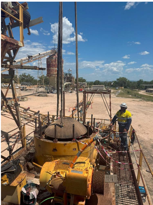
Area 01 removal of cone crusher mantle
