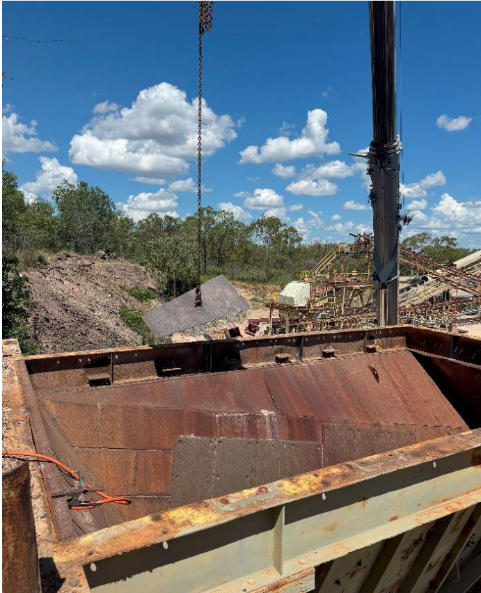
Bisalloy wear plate install for ROM repair
