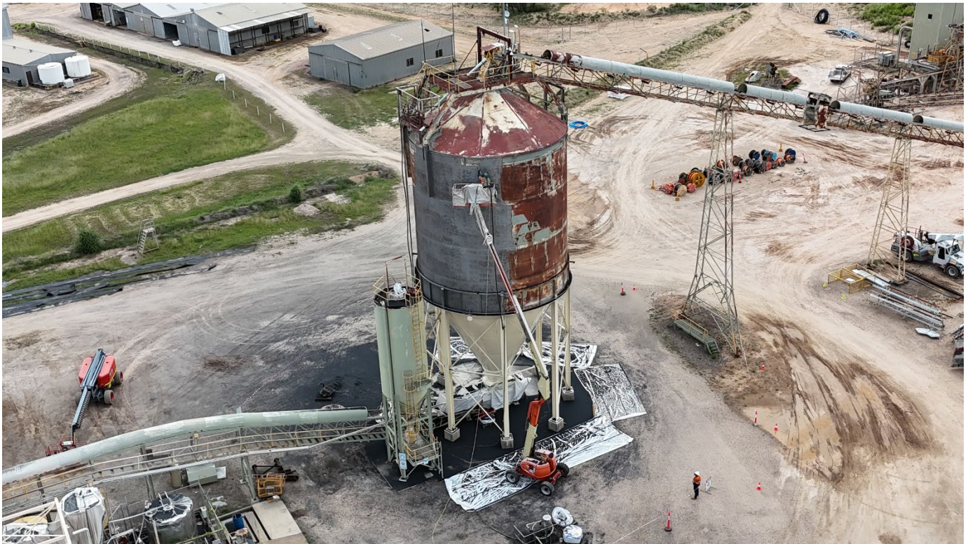
Blasting works at fine ore bin with lower section blasted and painted
