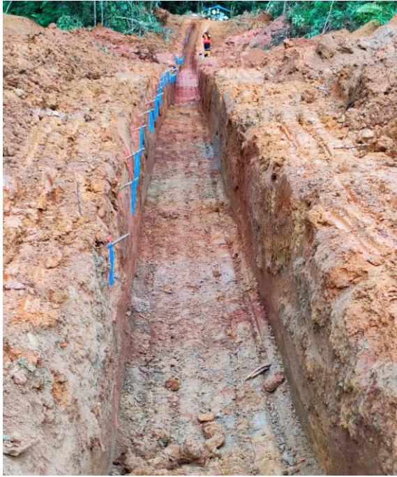
Little MacKenzie southern trench, with 2m sampling flagged ready for sampling.
